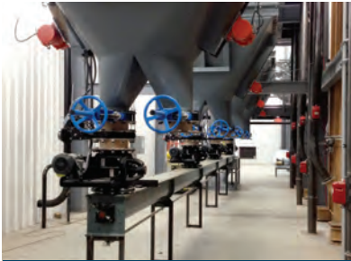
Inflatable Seat Butterfly Valve Overcomes Abrasive Material
