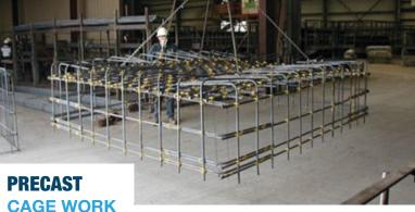
With Yellow 626 K-KLIPs, this cage is able to maintain its shape when free standing, eliminating the need for diagonal support bars and excessive wheel spacers.
