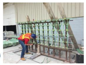
The Made in America (MIA) clips use recycled polycarbonate that won't crack, break, deform, rust or degrade, and they won't scratch or damage epoxy-coated rebar or fiberglass reinforcement either. Finally, each size is brightly colored to make them easy to distinguish and inspect. This system offers one of the fastest and safest ways of joining rebar without the need for wire or welding.
