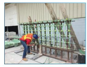
joints, or rebar to strand. The clips provide a four-point rigid grip that guarantees a tight, perfect connection every time. The Made in America (MIA) clips use recycled polycarbonate that won't crack, break, deform, rust or degrade, and they won't scratch or damage epoxy-coated rebar or fiberglass reinforce-ment either. Finally, each size is brightly colored to make them easy to distinguish and inspect.
