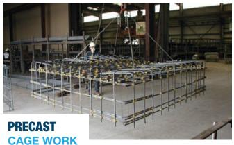
With Yellow 626 K-KLIPs, this cage is able to maintain its shape when free standing, eliminating the need for diagonal support bars and excessive wheel spacers.
