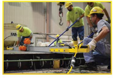
along the Form's rails as it strikes-off and straight-edges the concrete. Simultaneously, the Vibrators produce a downward centrifugal force of up to 1320 Lbf at 3600 vibrations-per-minute to both surface-finish, and consolidate the concrete to a depth of 12" to 18". The self-propelled feature provides two distinct advantages: **Safety** and **Speed**.
